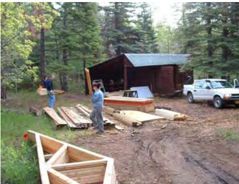
It starts with a pile of wood and some willing volunteers.
