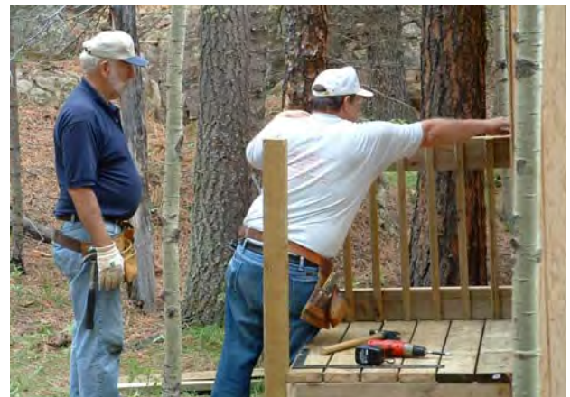
Larry showing Dan how to single-handedly plumb a wall.
